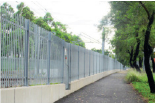
Homebush, Sydney. Rail corridor security fences should be robust, easily maintained, modular systems that are readily integrated with other urban design elements such as retaining walls.
