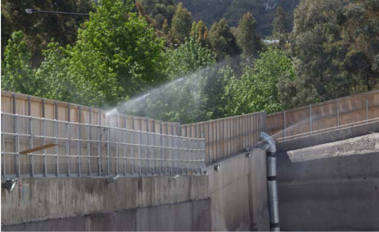
Figure 11 - Dust Mitigation at Norwest Station Site
