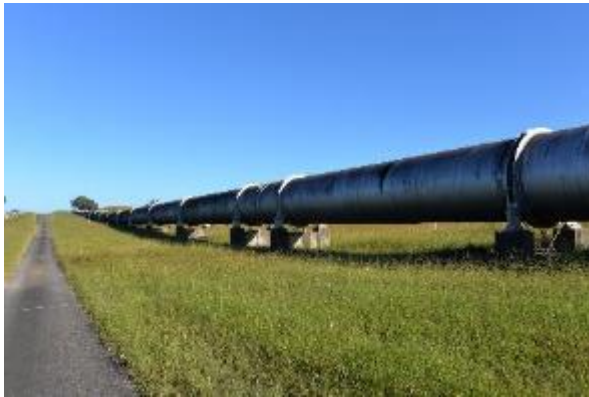
Figure 80. Pipe above natural ground level on concrete piers
