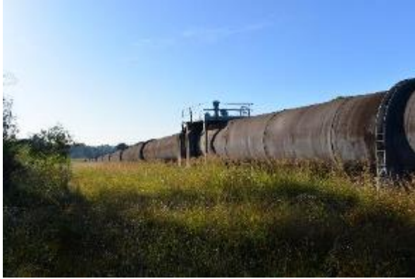
Figure 78. Pipeline and maintenance points
