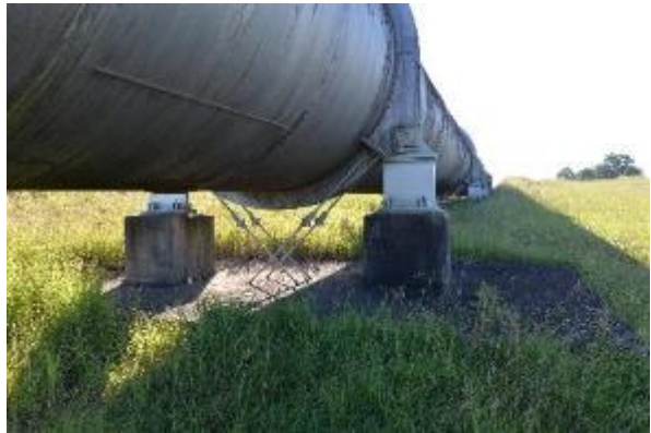
Figure 81. Detail of concrete piers and crossbeams
