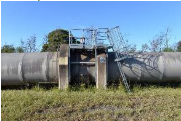
Figure 82. Maintenance/access point along pipeline
