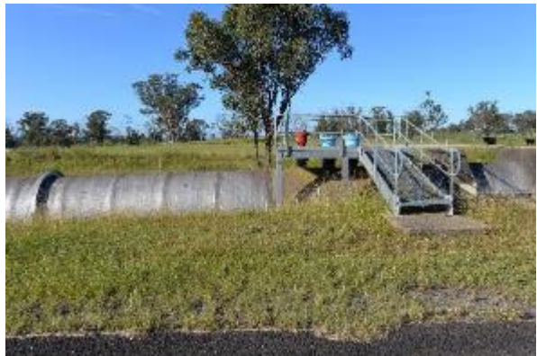
Figure 83. Maintenance/access ramp along pipeline
